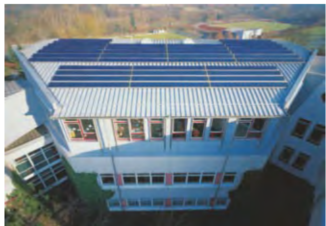
Project: Schiller School, Bretten, Germany Refurbishment project
