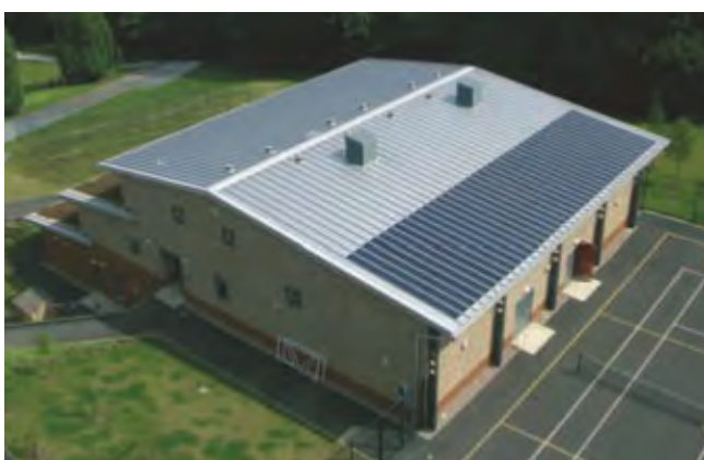
Project: Shrewsbury High School, Shropshire, UK Architect: The Girls Day School Trust
