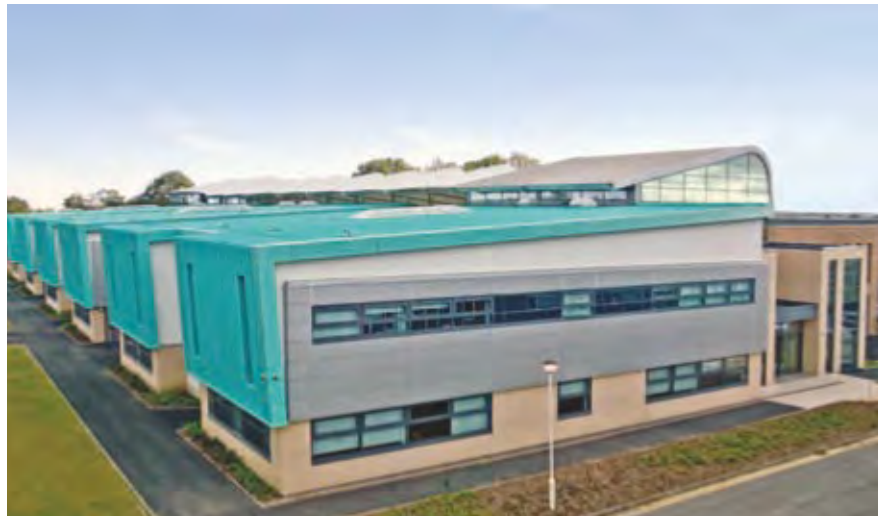
Project: Cramlington Junior Learning Village, Northumberland, UK Architect: Space Architecture
