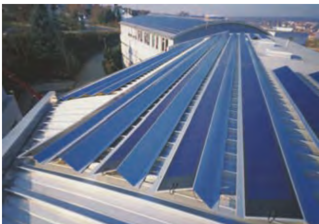
Project: Schiller School, Bretten, Germany Refurbishment project
