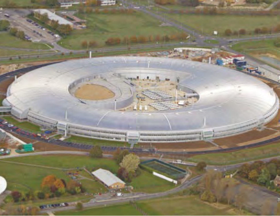
Project: Diamond Synchrotron, Didcot, UK Architect: Crispin Wride Architectural, Design Studio at Jacobs Engineering
