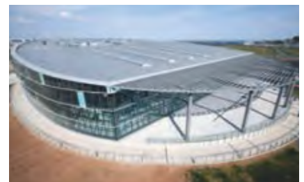
Project: Cardiff International Pool, Wales, UK Architect: S&P Architects
