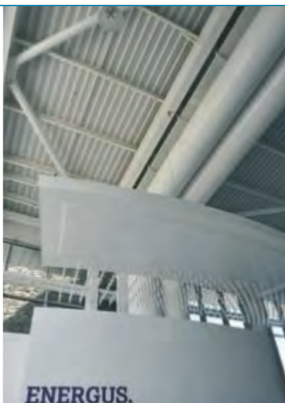
Project: Enerigus Centre of Excellence Workington, UK Architect: Plus (UK) Ltd
