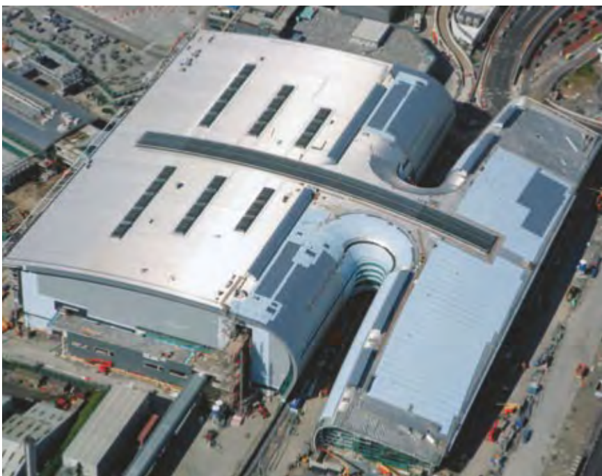
Project: Dublin Airport, Ireland Architect: Pascall+Watson
